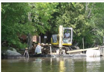
The Durant Dock is completely rebuilt.
