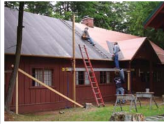
Workers apply waterproof underlayment to Spruce Dormitory roof.
